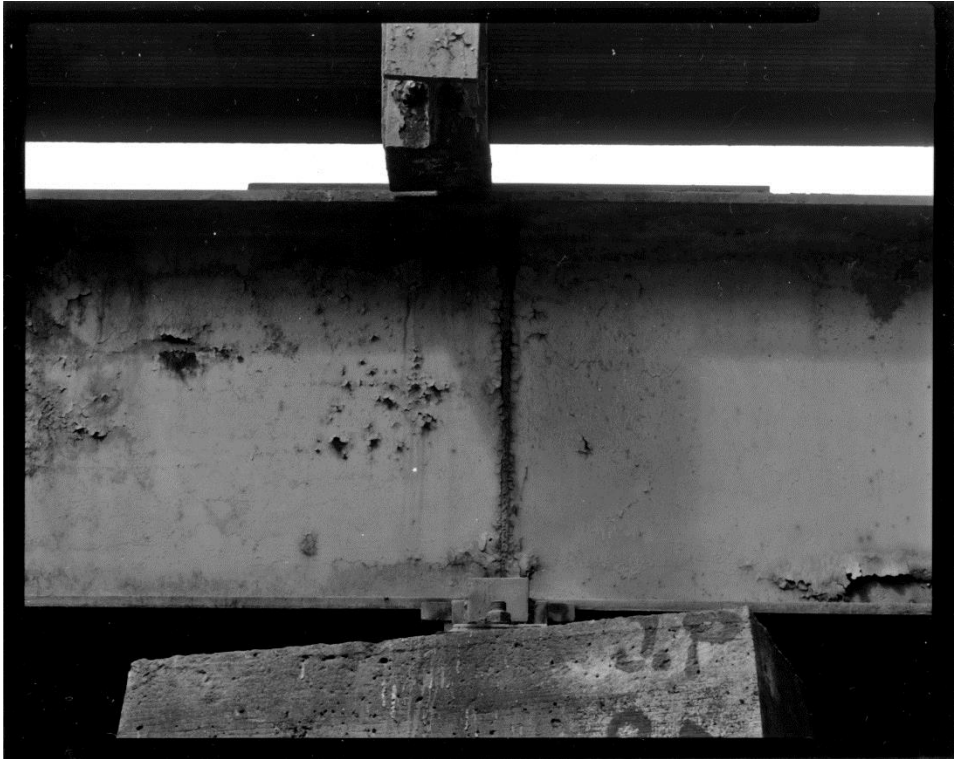
NH-744-11: Bearcamp River Bridge, bent 4, east side, showing detail of welded splice joint joining stringers over bent bearings, made to exact specifications to allow the stringers to function structurally as both simple and continuous beams. Looking northwest.
