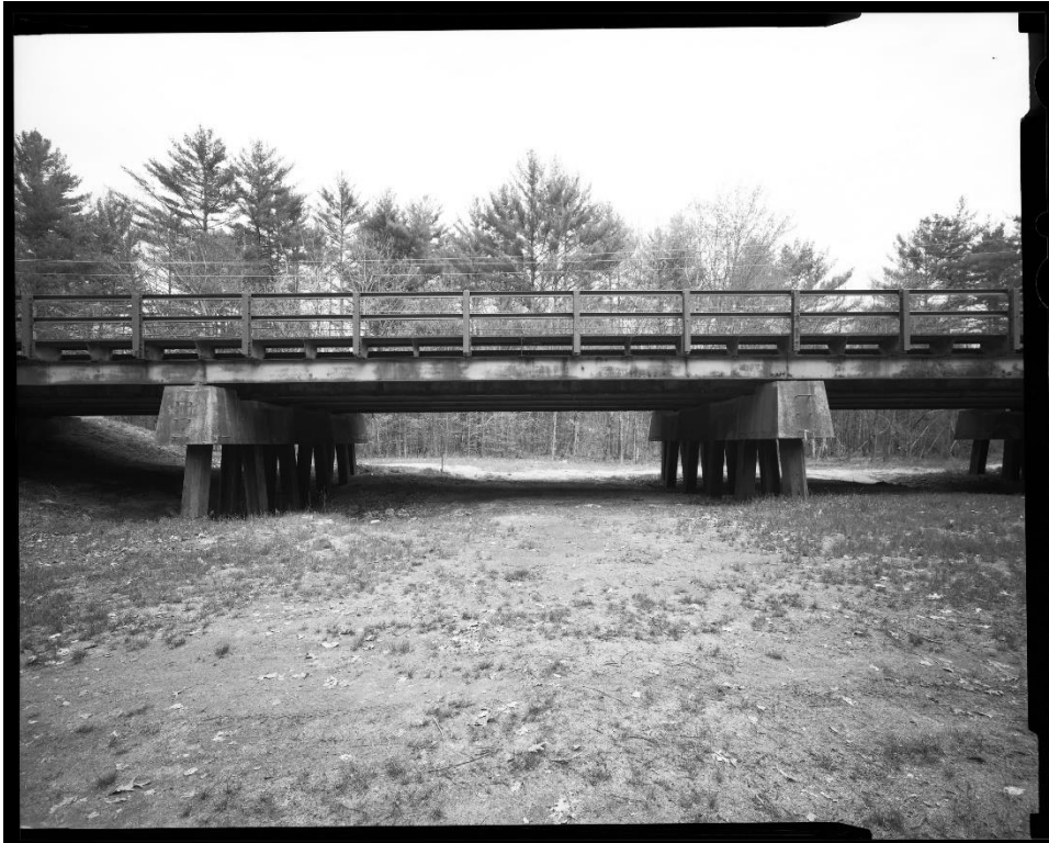
NH-744-15: Bearcamp River Relief Bridge, west (upstream) elevation showing bents 2 and 3. Looking southeast.
