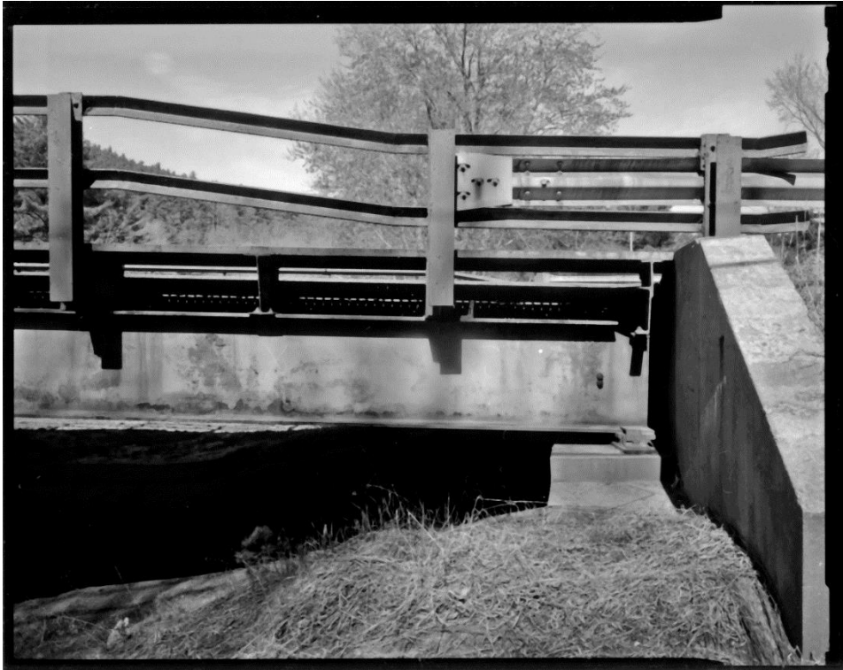
NH-744-10: Bearcamp River Bridge, north abutment, east side, showing abutment back wall, bearing, sidewalk assembly and railing. Looking northwest.
