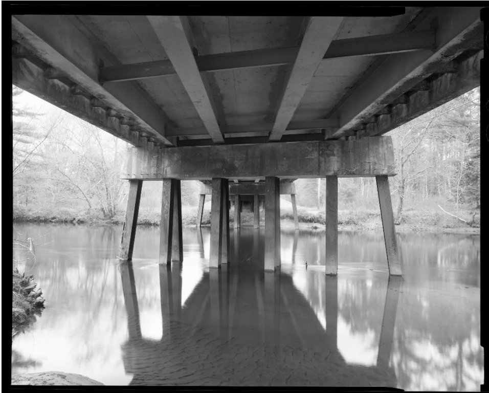
NH-744-7: Bearcamp River Bridge, bent 3, elevation, showing battered H-piles, concrete cap girder, rolled I-beam stringers with diaphragm bracing. Looking southwest.
