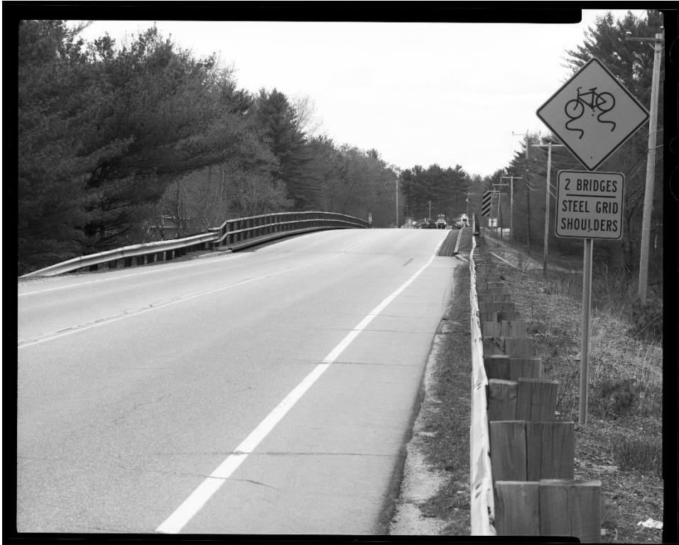
NH-744-1: Bearcamp River Bridge, south approach and view of deck showing slightly arched profile of superstructure most apparent in railing. Looking north.
