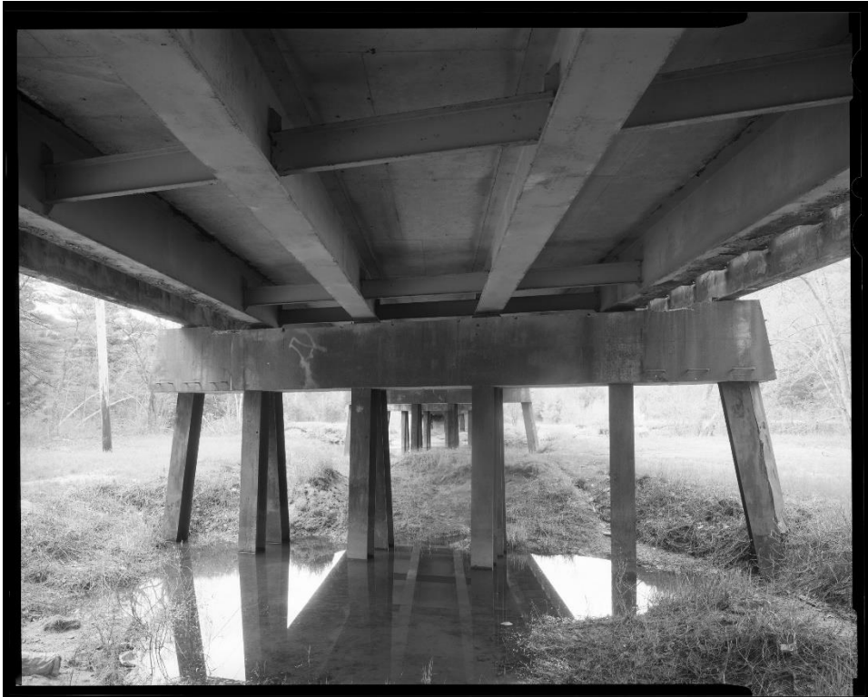
NH-744-6: Bearcamp River Bridge, bent 4, elevation, showing battered H-piles, concrete cap girder, rolled I-beam stringers with diaphragm bracing. Looking southwest.
