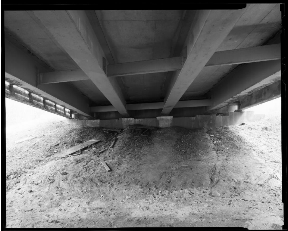
NH-744-8: Bearcamp River Bridge, north abutment elevation, showing rolled I-beam stringers with diaphragm bracing. Looking northeast.
