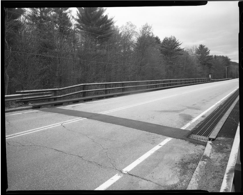
NH-744-16: Bearcamp River Relief Bridge, deck view, showing railing, open grate drains and expansion joint visible at right of asphalt patch. Looking south.
