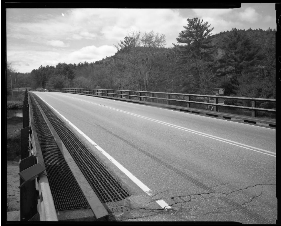
NH-744-5: Bearcamp River Bridge, north approach, view of deck showing steel grate curb drains and sidewalk. Looking southwest.
