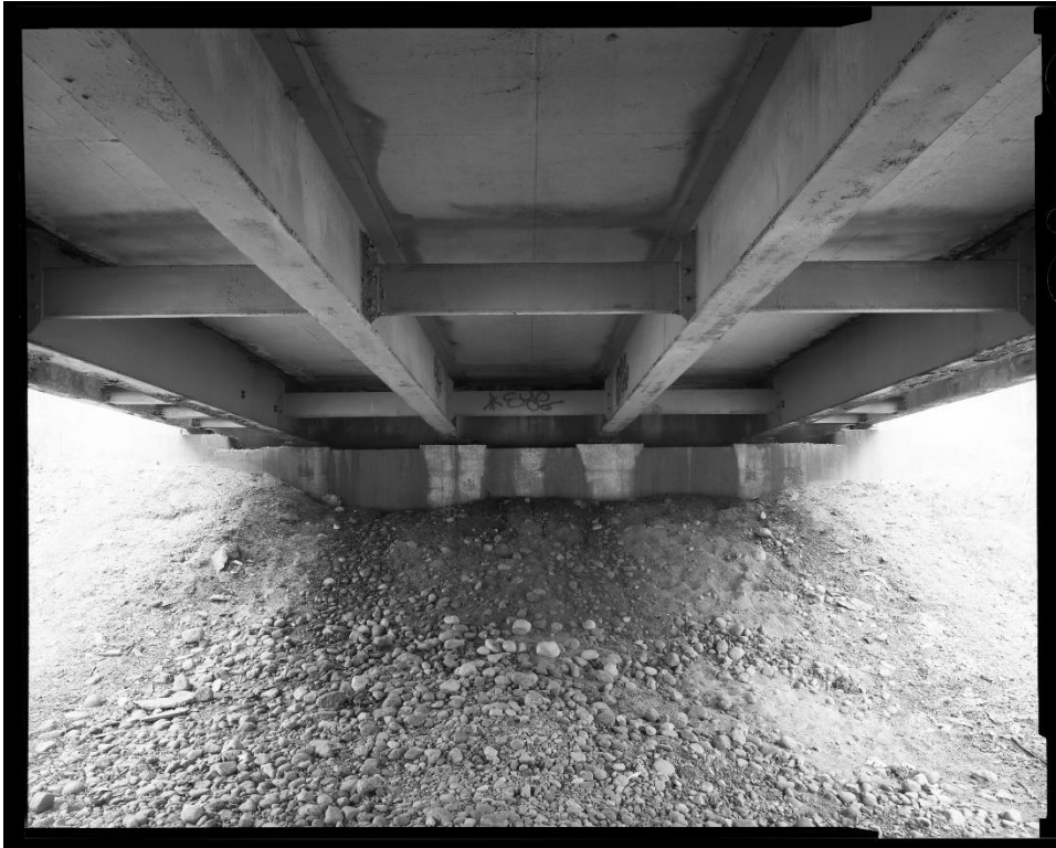
NH-744-18: Bearcamp River Relief Bridge, south abutment elevation, showing rolled I-beam stringers with diaphragm bracing. Looking southwest.
