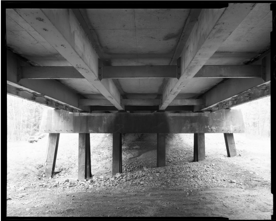
NH-744-17: Bearcamp River Relief Bridge, bent 1, and underside of deck showing stringers and diaphragms. Looking southwest.
