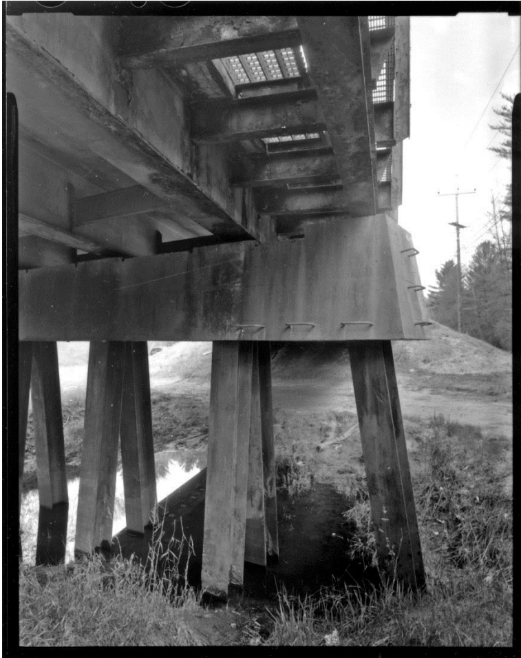
NH-744-9: Bearcamp River Bridge, bent 4, east side, showing battered H-piles, concrete cap girder equipped with flood-escape ladder rungs and the steel-grate sidewalk and curb assembly above. Looking northeast.
